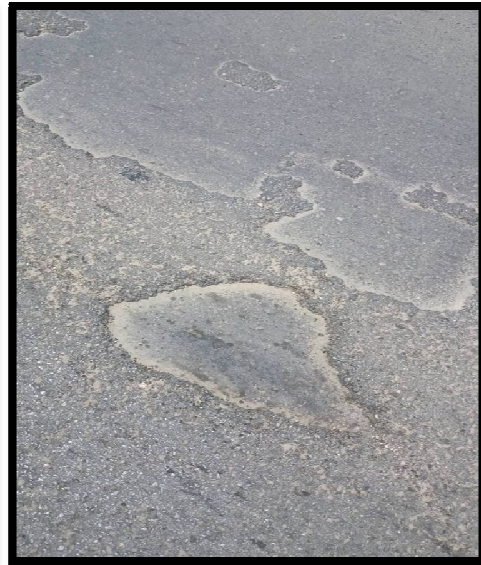
Figure III.35 : Arrachement
