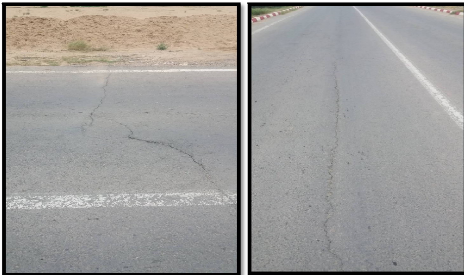
Figure III.32 : fissure transversal
