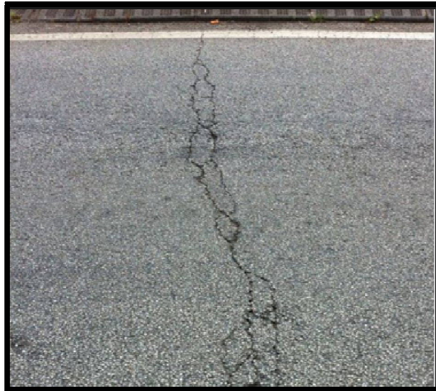
Figure II.19 : fissures transversales
