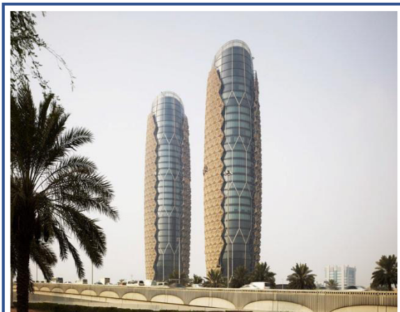
Figure 17 :Al Bhar tower Source : https://www.arch2o.com
