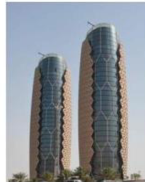
Figure 5: Al Bahar Towers.
