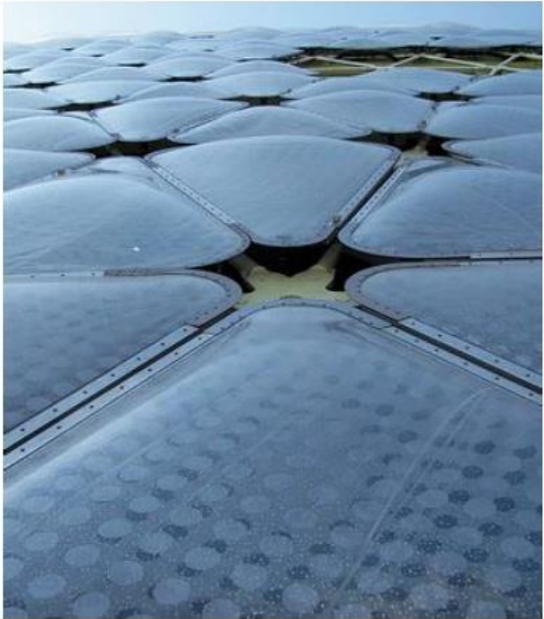
Figure 5: Detail of the inflating cushions
