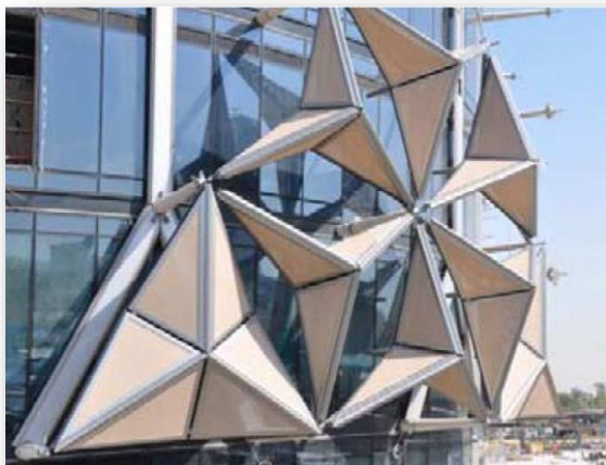
Fig.3: B Different possible configurations of the Al-Bahr façade system (Alotaibi, 2015)
