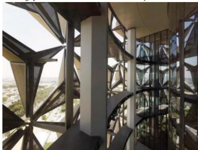
Figure 9: Inside view of the curtain wall system (Karanouh & Kerber, 2015)
