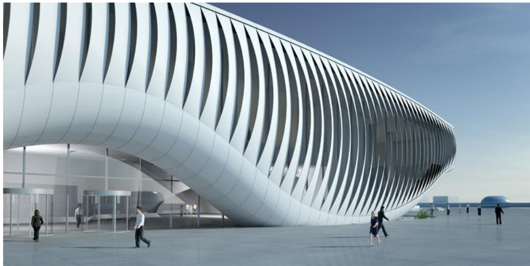
Figure 14: Lamellas in the façade
