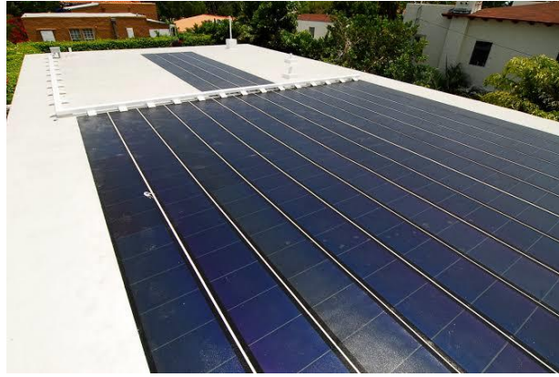
Figure I.9 : a-Si solar cell.
