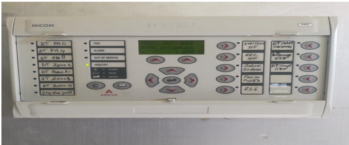
Fig.III.5 : Protection de distance (Micom P442)
