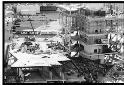
Figure 3-43 :Photo de musée pendant la construction. (Source : https://www.datumengineers.com/our-work/perot-museum-of-nature-and-science.html )
