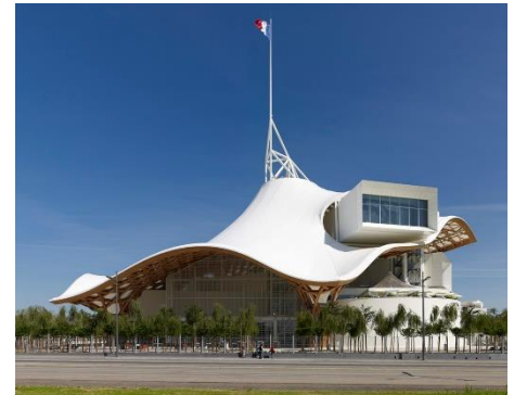
Picture 4-8 Centre Pompidou in Metz – Exterior. (©Didier Boy de la Tour, archdaily.com )
