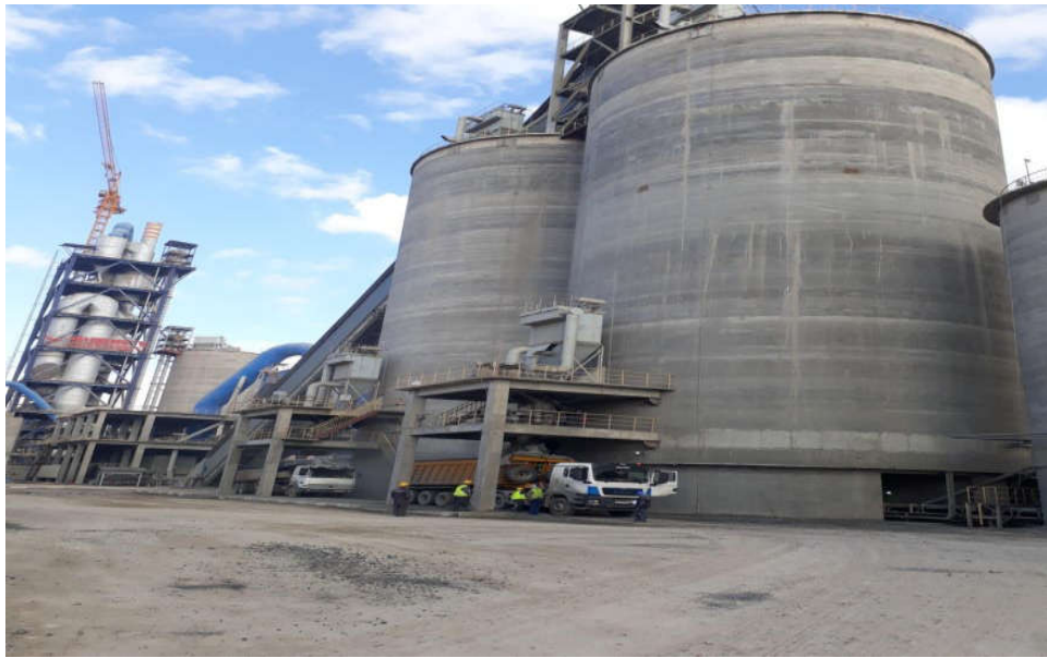
Figure I.12: Silos stockage de clinker.
