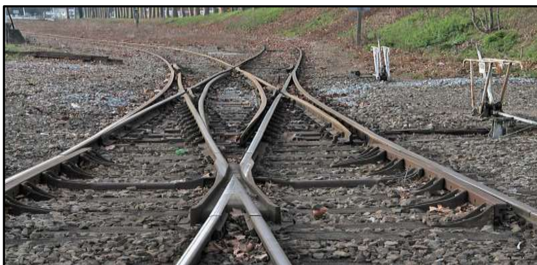
Figure 24 : Branchement Junction double
