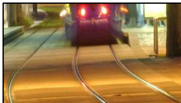
Figure 08 : rail tramway (gorge)
