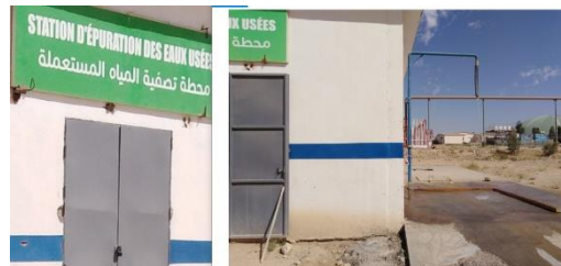
Figure II.12 : Station des eaux usées. [1]
