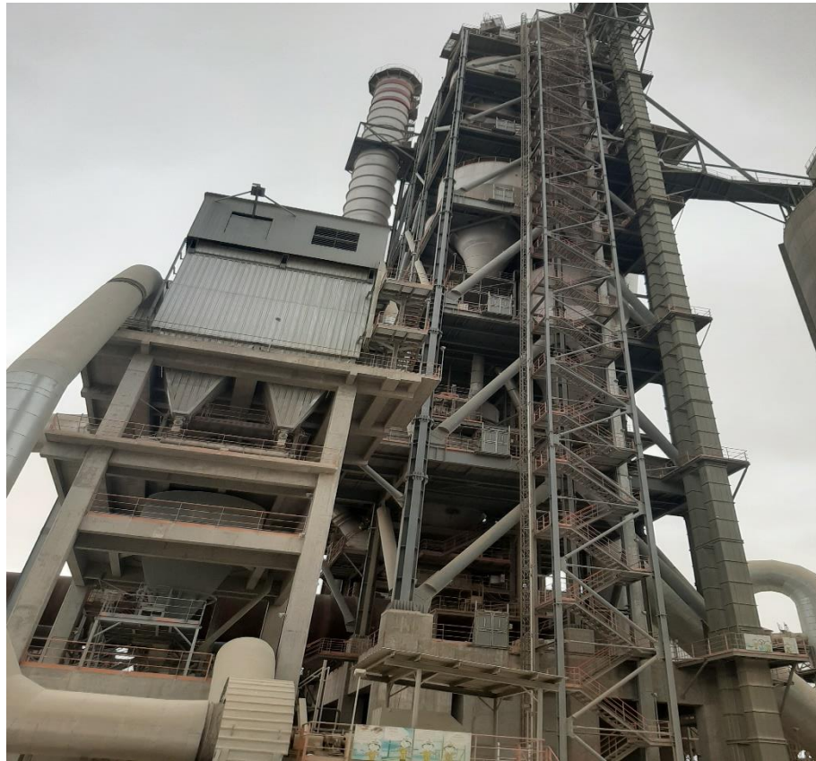
Figure I.11: Preheater or cyclones
