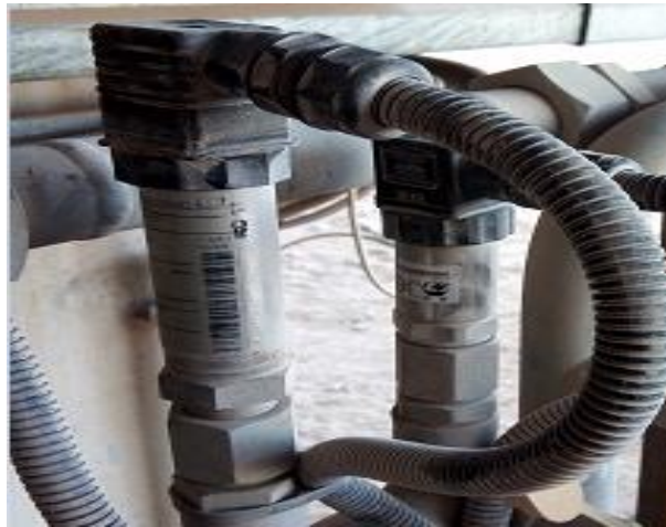
Figure III. 11: Capteur de pression.
