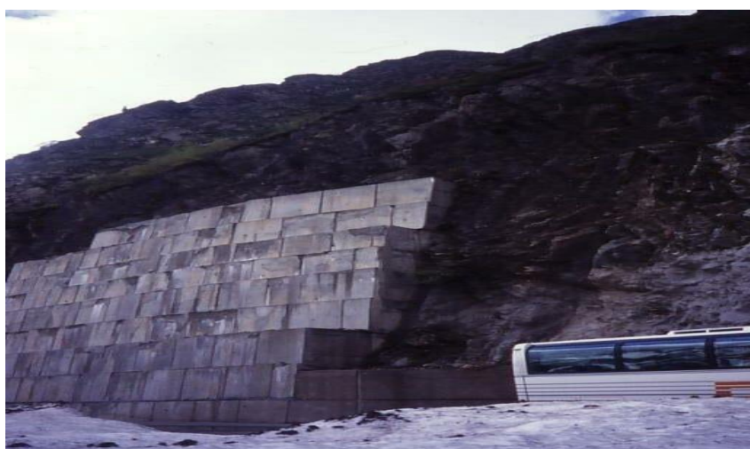
Figure II.1: Mur poids
