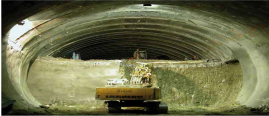
Figure II.6 : Creusement de demi-section.
