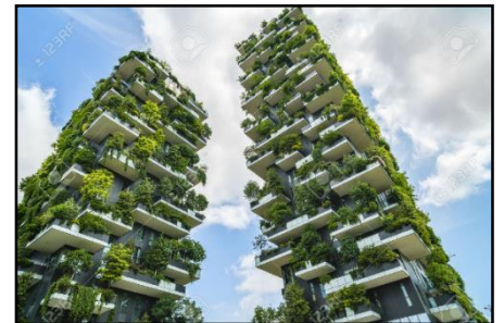
Figure 123 : Façade bosco verticale
