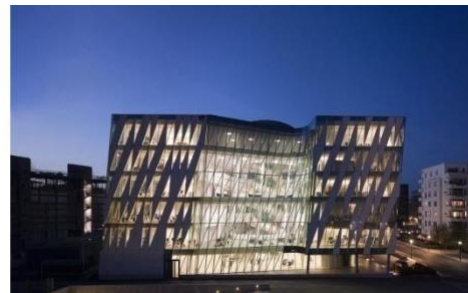
Figure 64: lights view de la banque saxo
