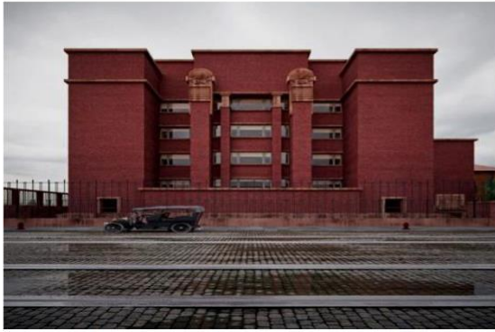
Figure 3: Larkin administration building 1906. Source: The Early Work of Frank Lloyd Wright: The "Ausgeführte Bauten" of 1911.
