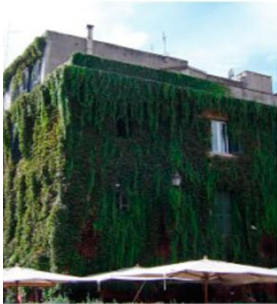
GREEN FACADE IN TRASTEVERE, ROME (ITALY)
