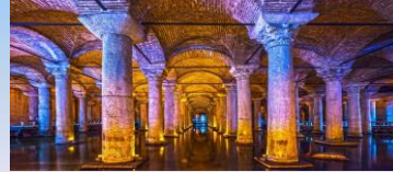
Romans built this huge water storage system underneath the city in 532. The cistern is supported by 336 columns and held enough water for the whole city to survive a long siege.
