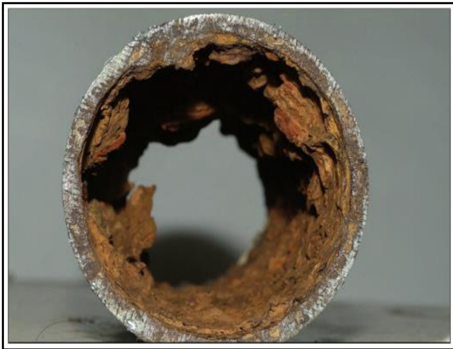
Figure I. 5: Microbial corrosion inside pipeline [29].
