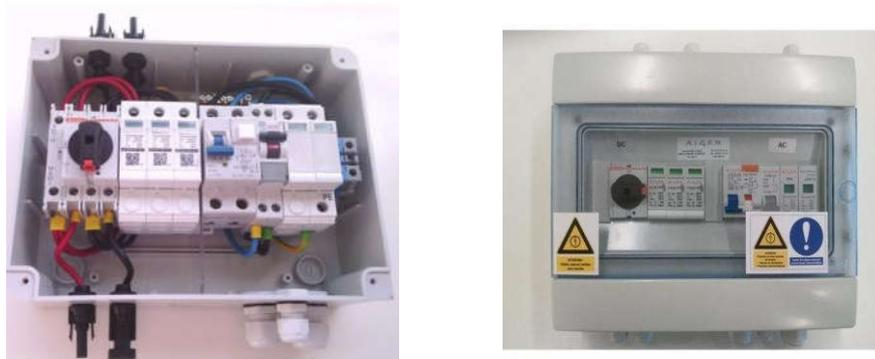
Figure 2-7 coffrets de protections photovoltaïques AC DC
