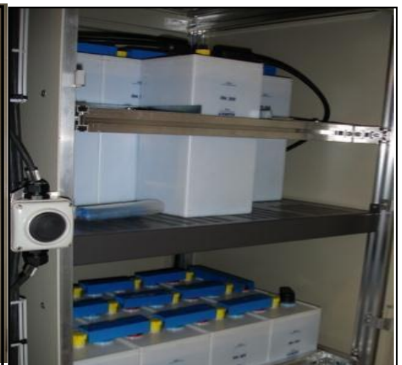
Figure IV.11 L'armoire des batteries24 V. [19]
