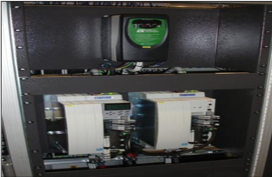
Figure IV.6 : Le tableau distribution 400 V.
