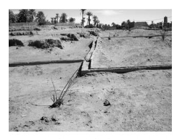
Fig. 16 A portion of the network of the foggara seguias El Méghier abandoned (photography Remini and Achour 2008)
