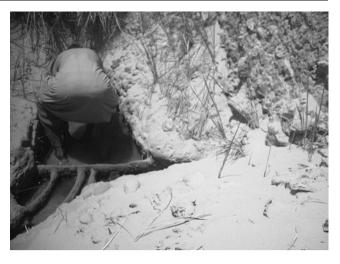
Fig. 17 A periodic cleaning of the foggara Kasria of Badou (photography Remini and Achour 2008)
