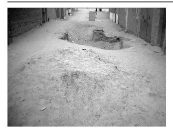
**Fig. 8** Collapse of a section of the gallery of the foggara Amokrane (Timimoun) during the flood of 2003 (photography Remini 2007)
