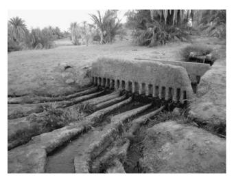
Fig. 3 The large comb (flow splitter) of the foggara El Meghier (Timimoun) (photography Remini and Achour 2008)
