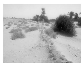
Fig. 18 Coverage of seguia by flat slabs of rock, a way to fight against sand (photography Remini 2007)
