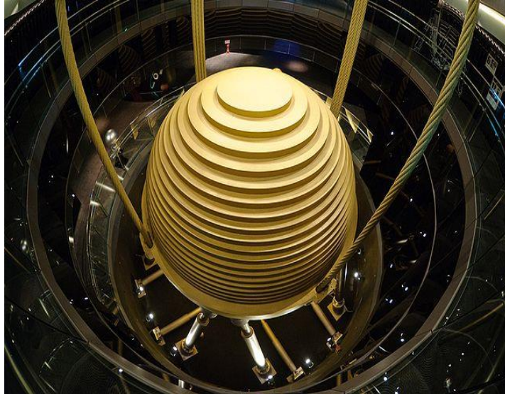
Figure 2.2 Tuned mass damper pendulaire de la tour Taipei 101
