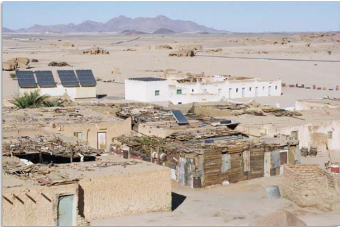
Figure 16: village in Tamanrasset powered by solar energy [ZOG 09]
