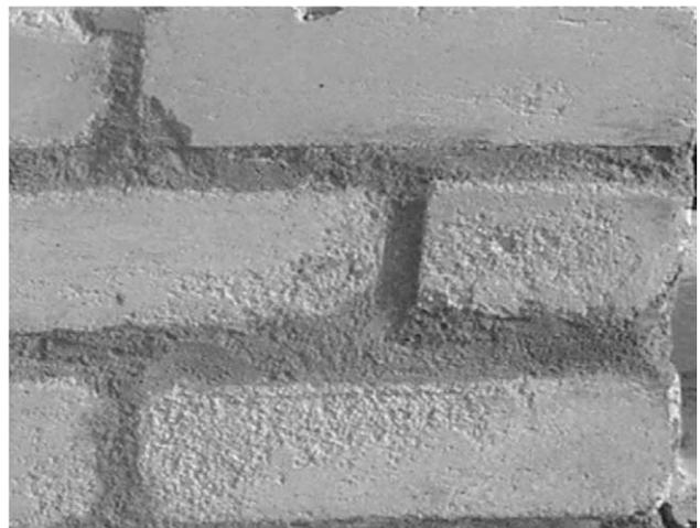
Fig. 9. 8% lime stabilized wall. Erosion deterioration after 48 months exposure.
