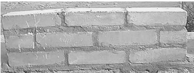
Fig. 11. 5% cement stabilized wall. After 48 months exposure.
