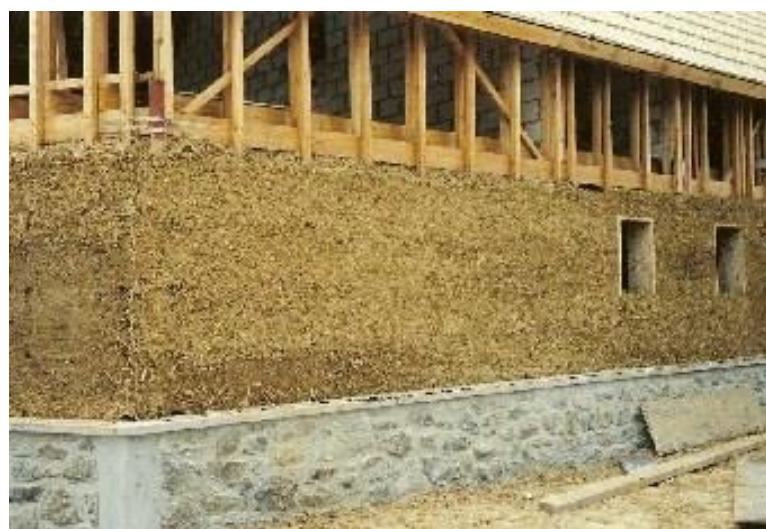
Figure 3-ch2 construction de mur terre-paille("mur terre-paille," www.google.com/url?sa=i&url=https%3A%2F%2Ffaisons-le-mur.com%2Fterre-paille 24/mai/2022.10h03)
