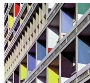
Figure II.30: avancé de façade, (Source Hegger, 2011)
