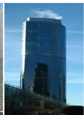
One wall Centre, Canada
