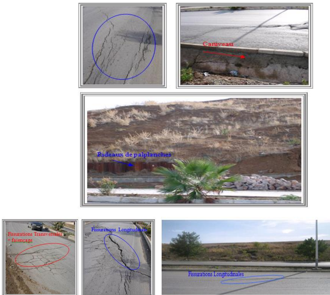
Figure 1.14 types des fissurations
