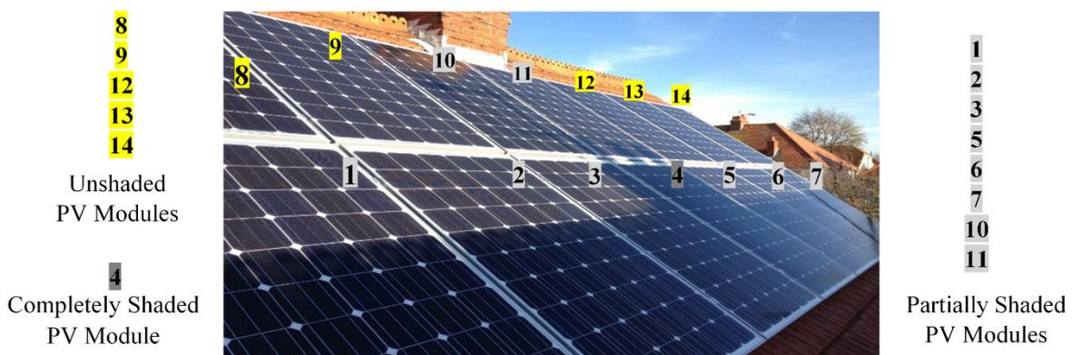
**Fig.IV.1.** PV array subject to shading conditions from an adjacent building [100]
