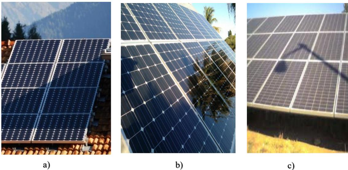
**Fig.II.1.** Shaded PV modules examples caused by a) nearby building elements
