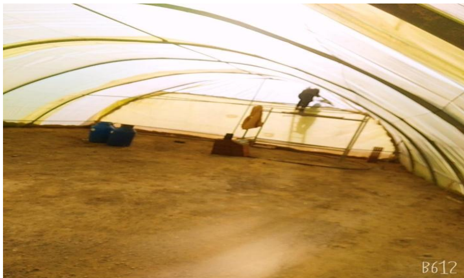
Figure 02: Installation of the greenhouse (Original)
