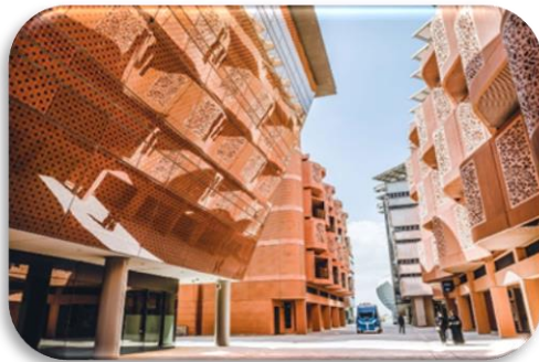
Figure 53 Sustainable materials in use at Masdar City (masdar news, 2023)
