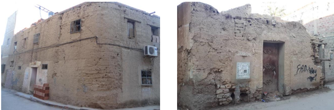
Figure 27: Vernacular house in M'cid neighborhood
