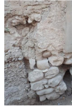
c/ the bedrock of house
