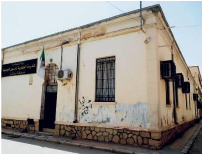
Figure 38: Colonial house made of local materials (earthen bricks, rocks, planks)
