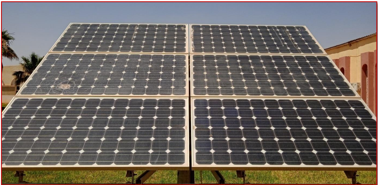
Figure 2: Installation panneaux solaire . (7)
