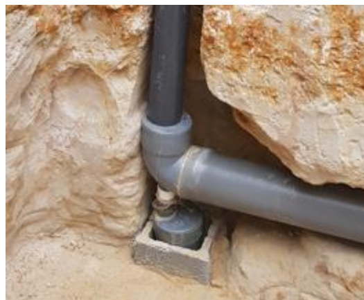
Figure II.10 Condensate drainage system.
