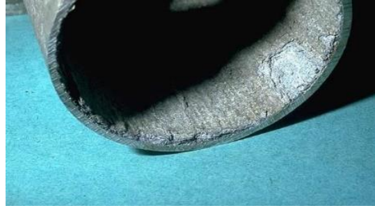
Fig I.5: Intergranular corrosion of metal
