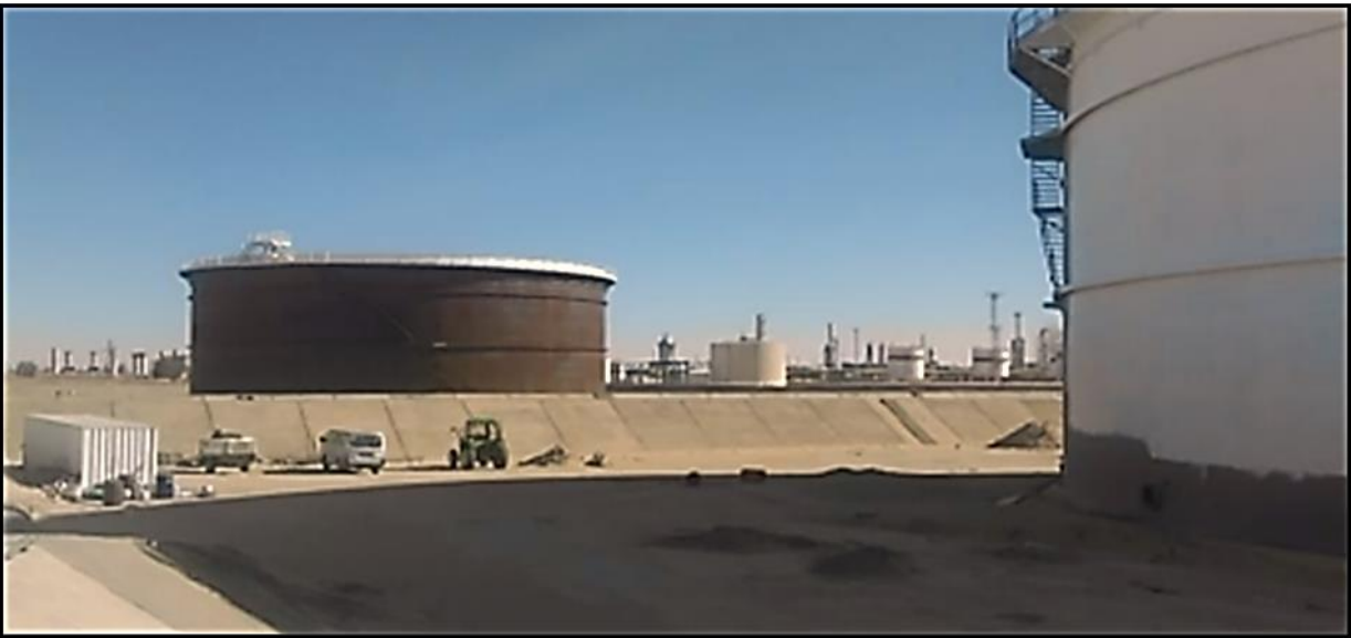
Figure 9: fuel storage Sonatrach, Hassi-Messaoud
