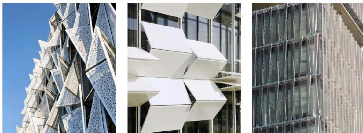
a) b) c) Fig. 17: Some pictures of kinetic façades: a) Campus Kolding, Kolding (Denmark), 2014; b) Kiefer Technic Showroom, Bad Gleichen Berg (A), 2007; c) ThyssenKrupp Quarter, Essen (DE), 2010
