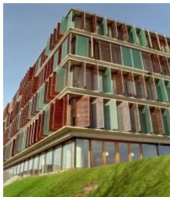
Figure 13: Rotating vertical fins: robotics and mechatronics center by Birk Heilmeyer and Frenzel Architects, Weßling, Germany Source: https://co.pinterest.com
