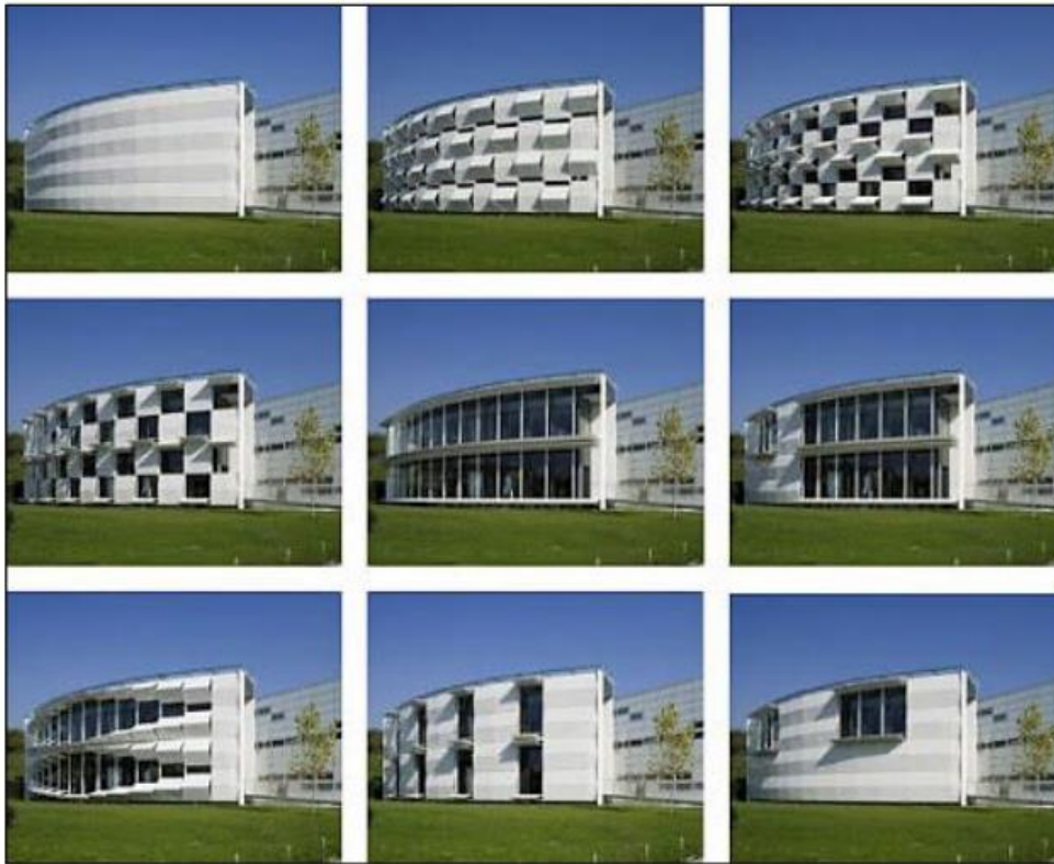
Figure 35: The kinetic system of the KIEFER Technic Showroom facade. (The different scenarios). (Source http://www.salazarposada.com/es/blog/detalle/blog-40 ).
