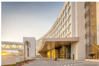
Figure 84: Hôtel Hyatt Regency Algiers Airport
