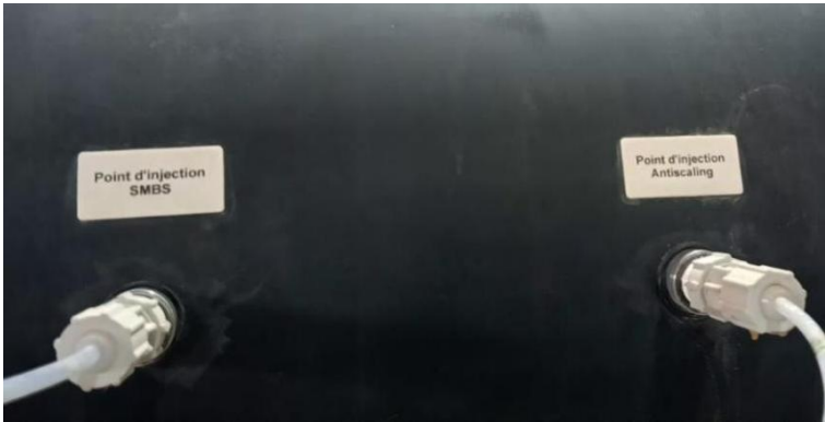
Figure III.26. Injection points
