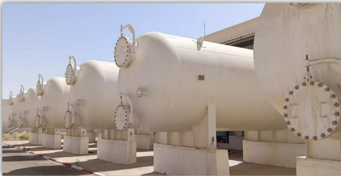
Figure III.22. Sand filters
