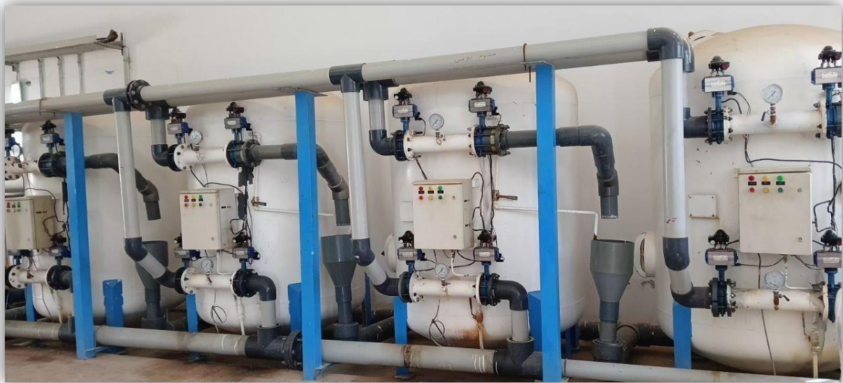
Figure III.5. Sand filters
