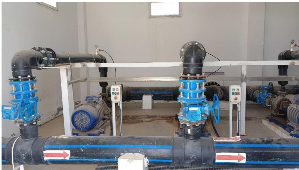
Figure III.32. Discharge pumps
