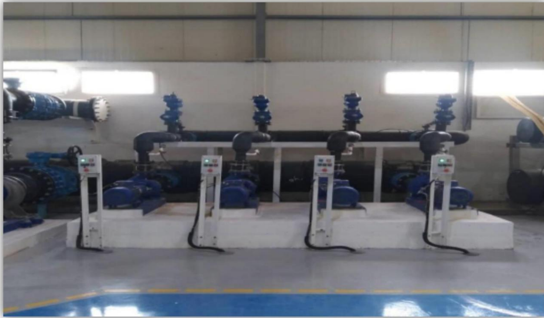
Figure III.23. Mixing pumps
