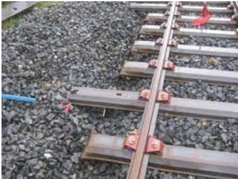
Figure 25 : System for fixing rails to metal sleepers.
