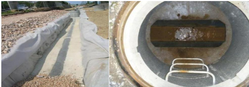
Figure 34 : Photo of a CD before installation of draining materials
