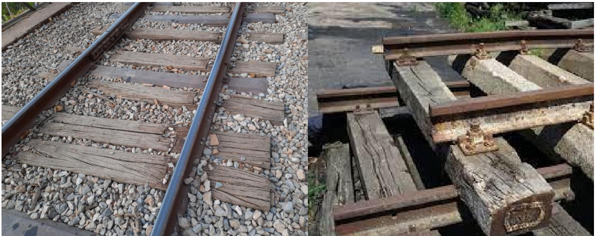
Figure 13 : Model of a wooden sleeper.
