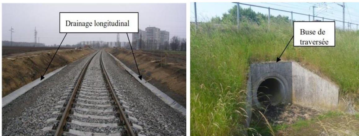
Figure 31 : Longitudinal and transverse drainage of railway tracks
