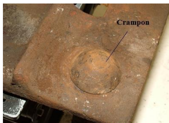
Figure 17 : Top view of the head of a crampon with a rounded section.
