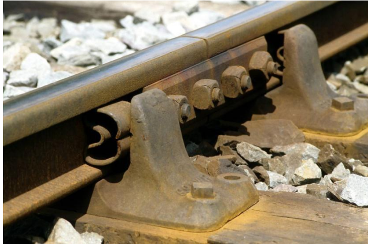
Figure 24 : System for fixing rails to wooden sleepers.
