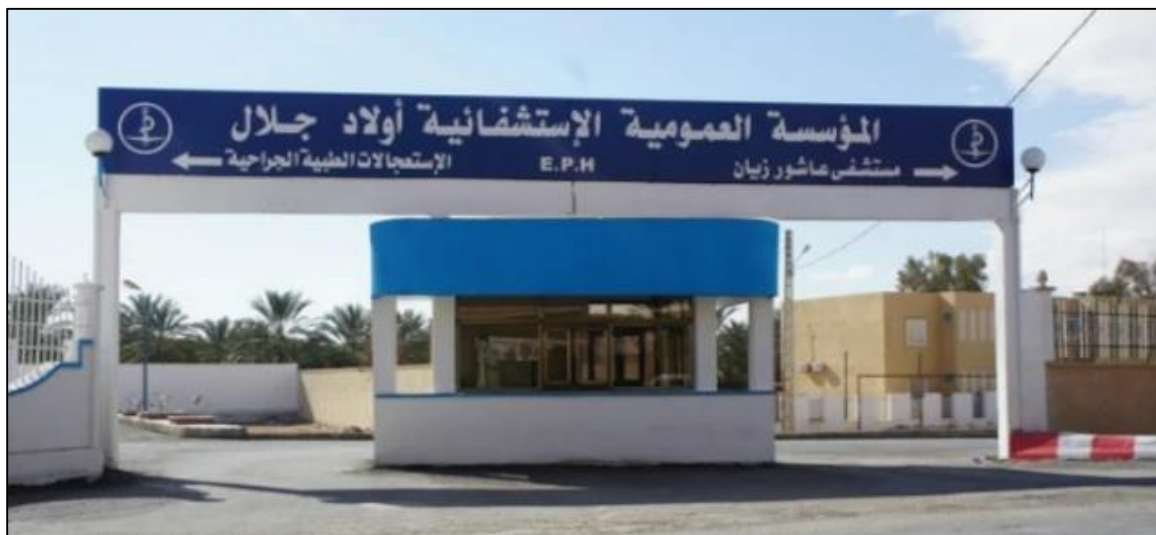
Figure 6. Photo d'Hôpital Achour Ziane de Ouled djellal (site web 5).
