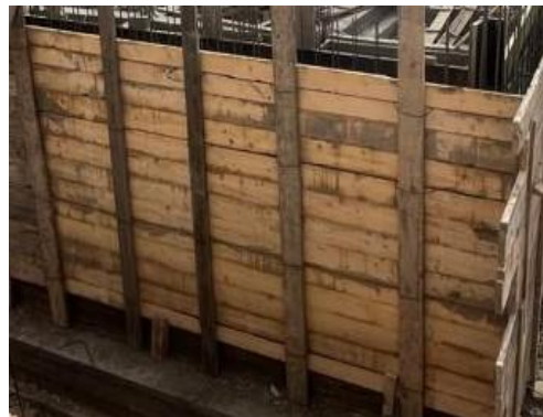
Figure.1.38. Assurer le coffrage.
