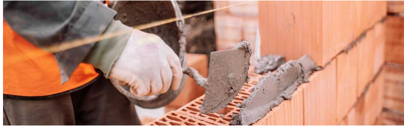
Figure I.6 : Pose de mortier de hourdage. [22]
