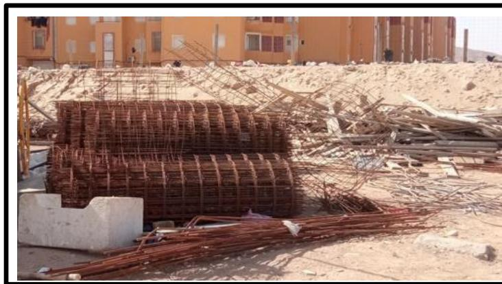
**Figure 1.15.** Treillis soudé
