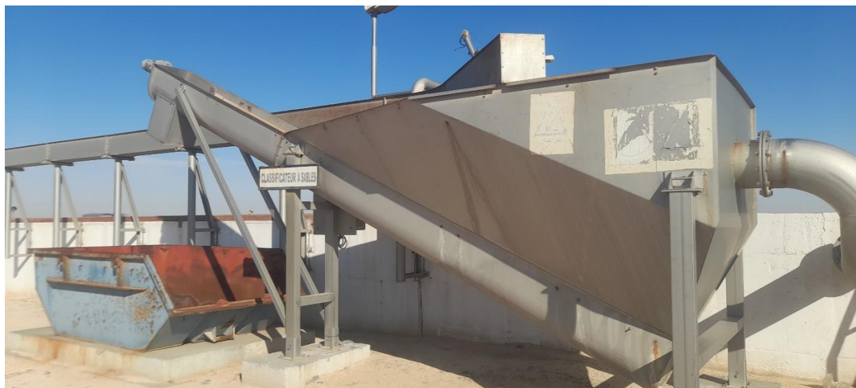
Figure I.3 : Dessablage [STEP KOUININE]
