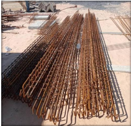
FIGURE 1.13: stockage des ferrailages
