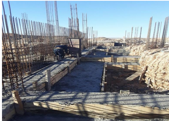
Figure 22. Pouring of foundation concrete (Source: Author, 2025).
