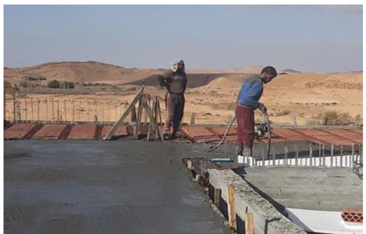
Figure 28. Casting of the first floor slab concrete (Source: Author, 2025).
