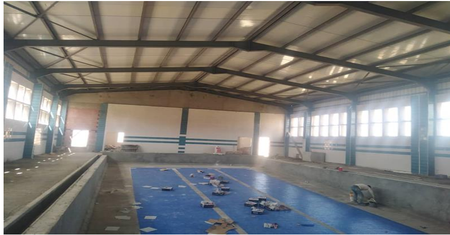
Figure 38. Covering of the metallic structure of the swimming pool roof (Source: Author, 2025).
