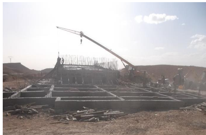
Figure 23. Casting of foundation column concrete elements (Source: Author, 2025).
