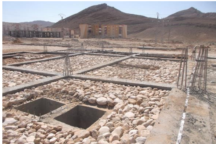
Figure 24. Placement of insulating stones for the ground layer (Source: Author, 2025).
