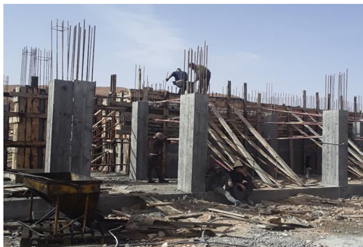
Figure 25. Casting of ground floor column concrete (Source: Author, 2025).
