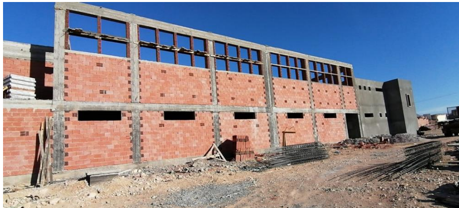
Figure 33. Setting out and defining the lighting openings on the first floor (Source: Author, 2025).
