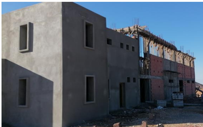
Figure 31. Progress of exterior plastering works on the first floor walls (Source: Author, 2025).
