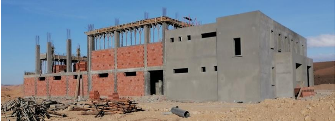
Figure 31. Execution of brick wall construction and plastering for the first floor (Source: Author, 2025).
