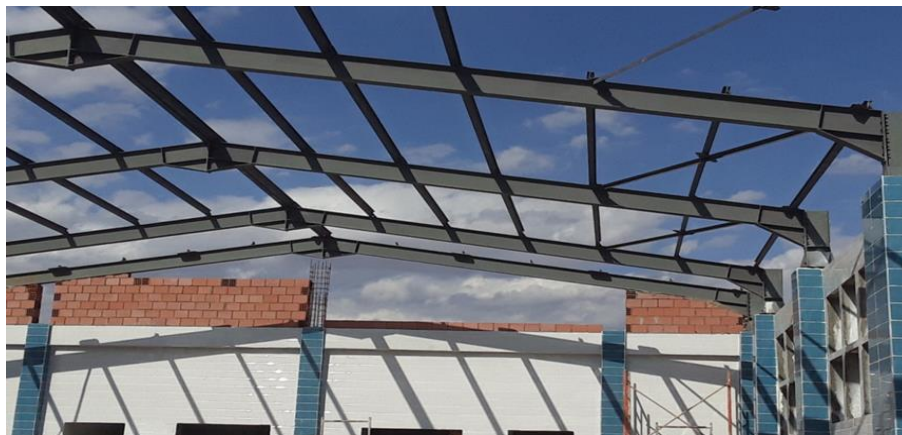
Figure 37. Installation of the metallic structure for the swimming pool roof (Source: Author, 2025).
