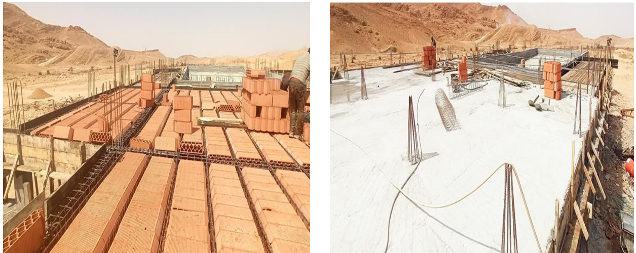
Figure 26. Start of concrete casting for the ground floor slab (Source: Author, 2025).
