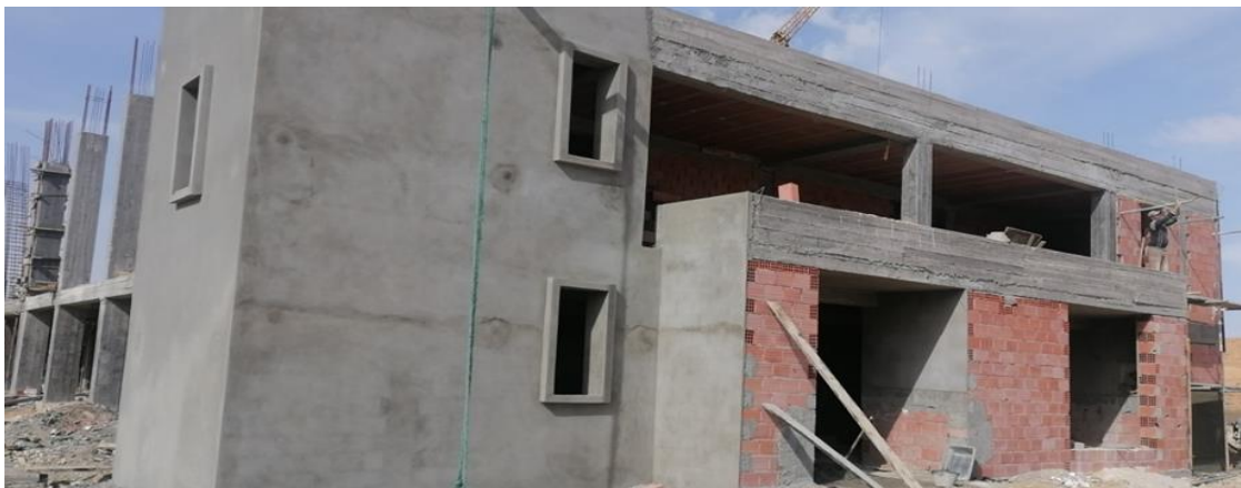
Figure 30. Cement plastering works on the first floor walls (Source: Author, 2025).
