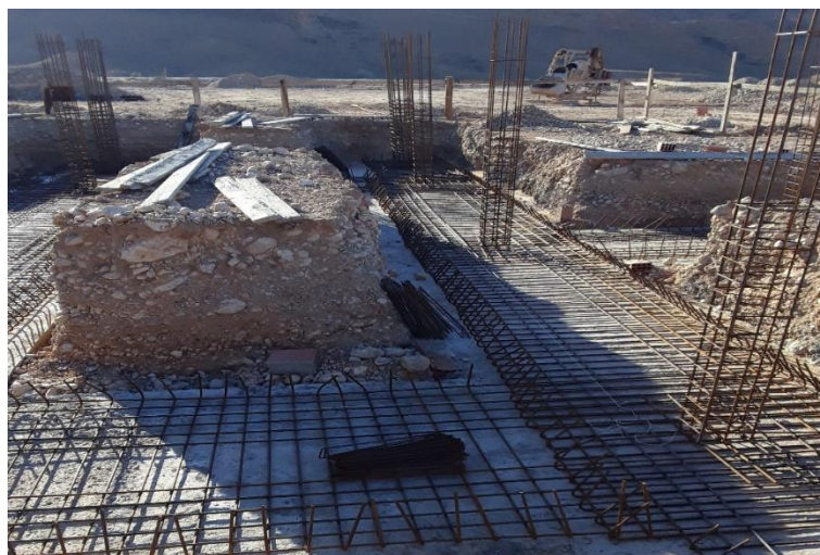
Figure 21. Placement of foundation reinforcement (Source: Author, 2025).
