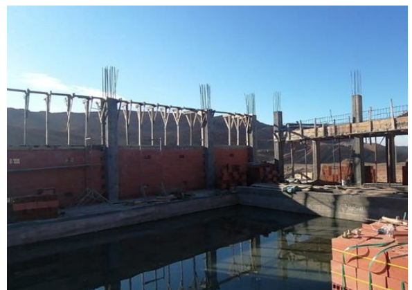
Figure 32. Water filling of the swimming pool basin for testing and commissioning (Source: Author, 2025).
