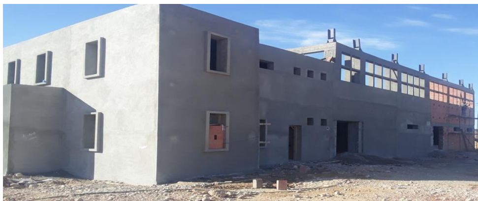
Figure 34. Exterior view showing the completion of first floor wall plastering and lighting window openings (Source: Author, 2025).
