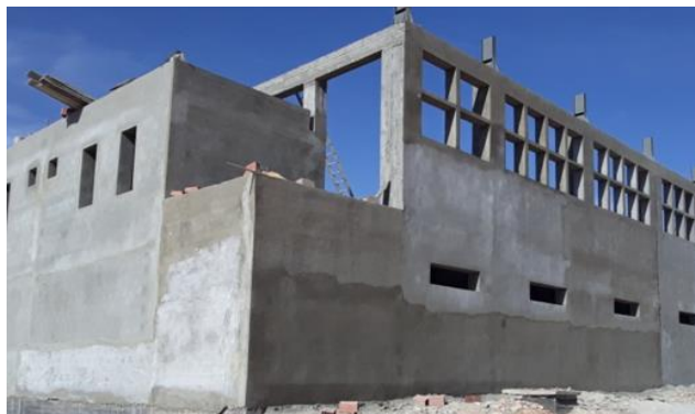
Figure 35. Execution of full exterior cement plastering works on the building façade (Source: Author, 2025).
