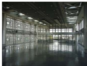
Figure 196: The effect of this opening on the distribution of natural lighting in the spaces of the institute
