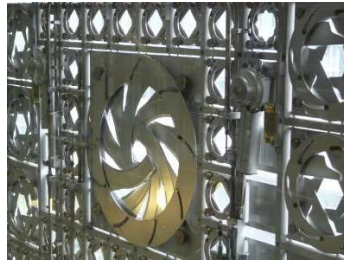
Figure 193: The shape of the facade from the outside when the diaphragms are closed
