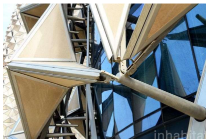
Figure 219: Independent Support Frame up close
