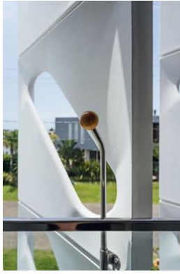
Figure 99: Rotatable GRC unit to allow for open views and ventilation
